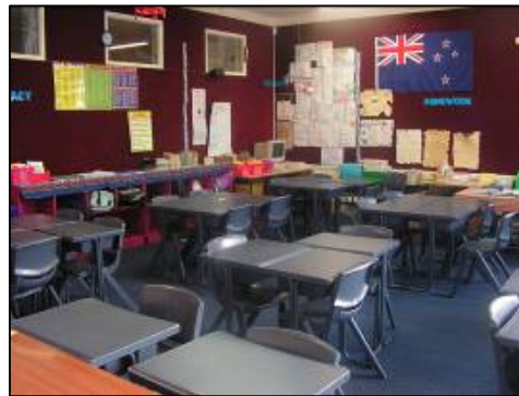
Refurbished classroom with new carpet and sound reducing pin-board wall lining.
